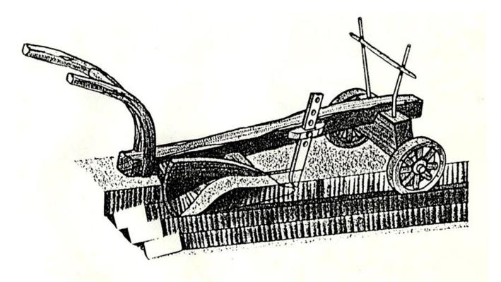
The plough has wheels on the front, so that it could easily be taken from field to field. The major innovation lies in the way the plough cuts. On the frame ahead of the share is a knife, placed vertically to cut the sod and make it easier for the share to enter the thick soil. Behind the share is a curved, wing-like board, sitting diagonally to the frame, to lift the cut sod and throw it clear to the right, like a wave
